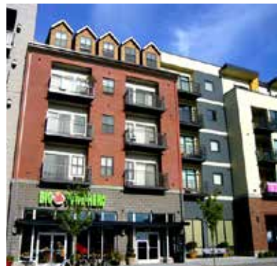
An example of an excessive number of colors and materials on one facade
