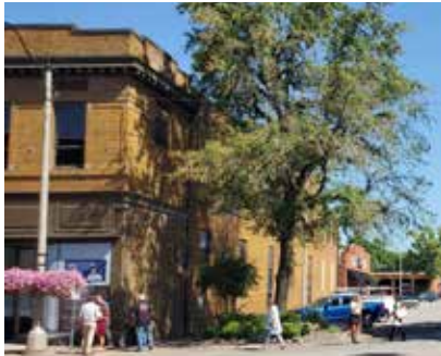
An example of a well-executed corner return in downtown Sapulpa
