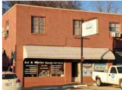
Inappropriate signage, lighting, and awnings
