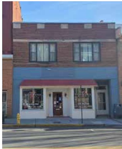
Example of inappropriate bulkheads and windows
