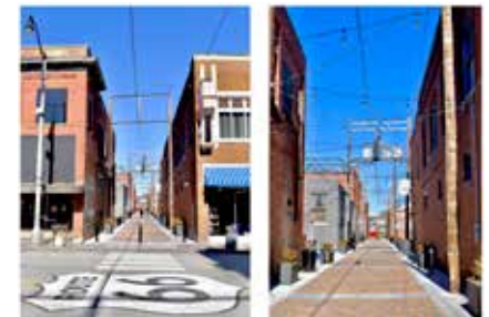
The new Alley District
